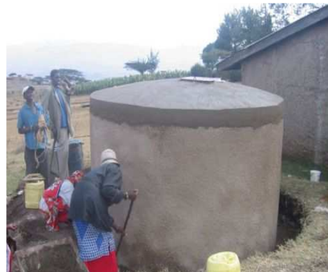
Figure 2: RWH Tank being built in Oleopolis vilage (funded by Ryan’s Well)
